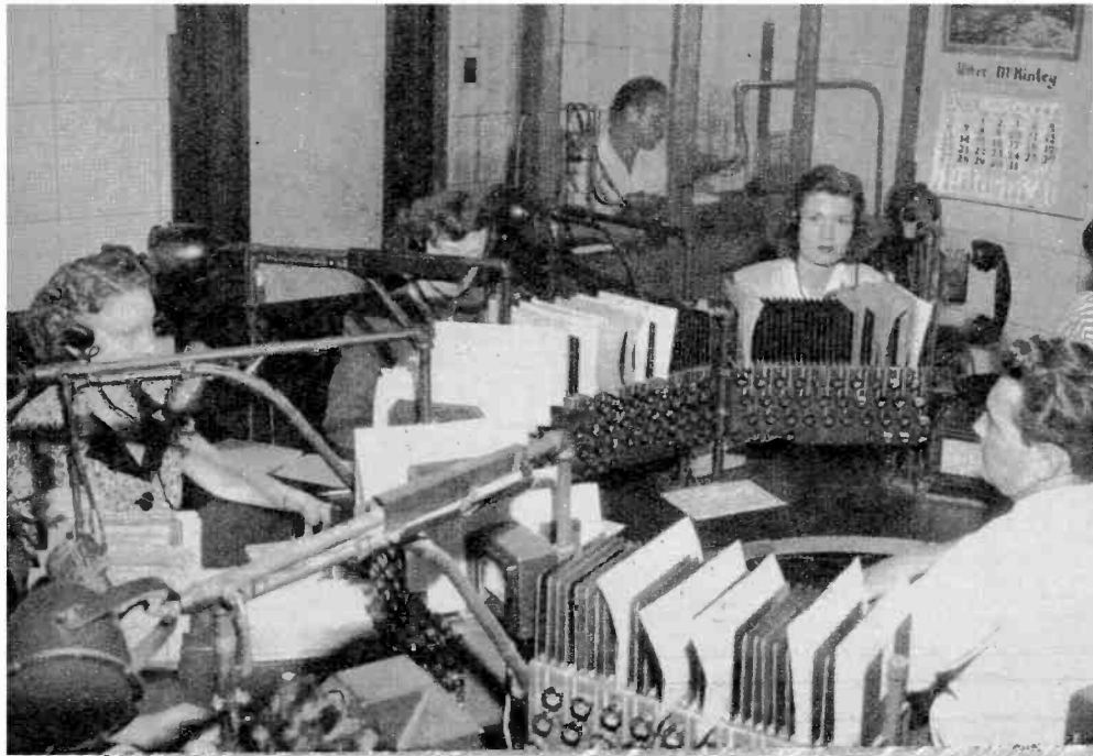
◀ COMMUNICATIONS ROOM OF KGPL shows radio operators seated around semi-circular table with monitor in background and dispatching supervisor at extreme right. Girls work in eight-hour shifts.
